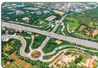
Outer Ring Road TGPA Junction
